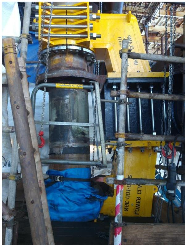
Figure 4: Neptune-engineered double-clamp system successfully installed onto the producing gas riser.
